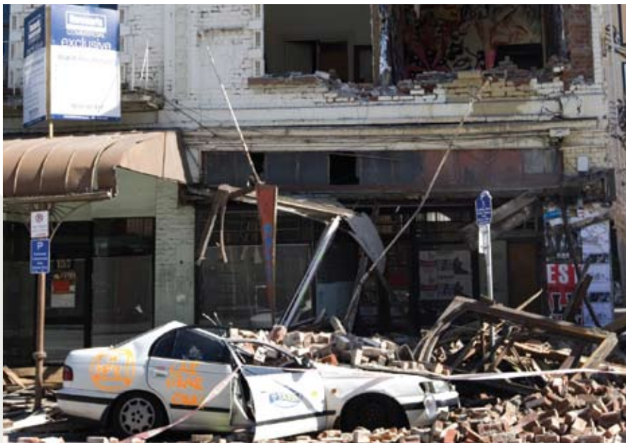
A taxi crushed by falling debris on Lichfield Street, Christchurch CBD.
